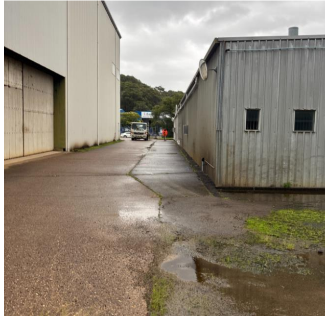
Photo 2 Existing site sheds, facing west
