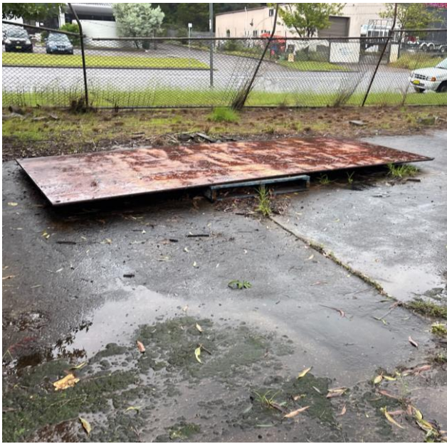
Photo 5 Metal sheeting at rear of site
