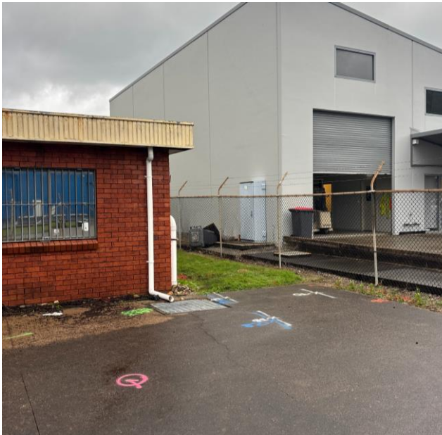
Photo 7 Pavement condition at front of site
