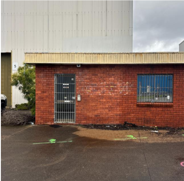
Photo 1 Existing building at front of site, facing east
